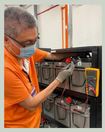
Integrated Supervisory Control System network enables the Power Facilities Regulator to monitor the battery's health condition remotely and accurately. This enables early detection of batteries with high temperatures so that they can be rectified immediately, to minimise the risk of fire and loss of backup power supply.
