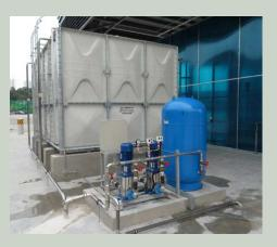
with automated bus washing machines that are fitted with an underground water recycling system to collect, filter and recycle about 80% of the water used in the washing process. The first rinse uses filtered recycled water while the final rinse uses clean water which is then drained back to an underground storage tank for filtration and reuse.
